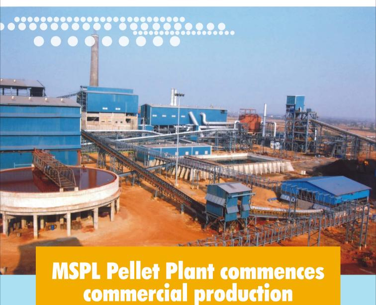
In July 2009, the Baldota group laid the foundation stone for MSPL Pellet Plant as part of its strategic forward integration plan. In 18 months the plant with a capacity of 1.2 MTPA was commissioned and commenced commercial production. Built at an investment of nearly 300 crores, the pellet plant is modeled on the Grate-Kiln Technology which enables production of high quality pellets at the lowest possible cost.
