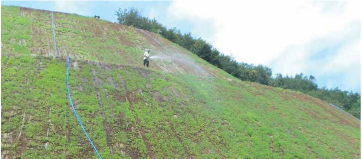
Geo-textile work being done on the slope of the dump to develop a green belt at PVS Mine as part of the Reclamation & Rehabilitation project.
