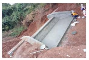
Among the artificial rain water harvesting mechanisms, check dams have received considerable importance in India as well as the other countries. Check dams are small barriers built across the direction of water flow such as channel, stream, nala, etc., to capture the rain water.
